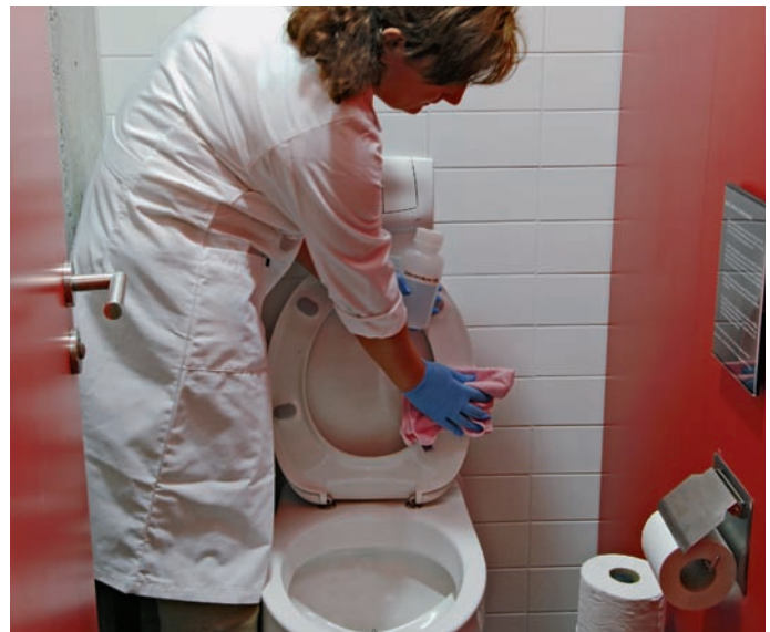
The right mixture: To clean NoMix toilets without contaminating the urine, one can use a 10 % citric acid solution and a microfibre cloth (Photo Ruedi Keller)
